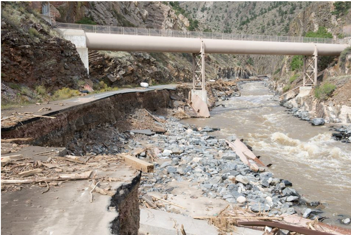
Figure 10: Extreme rainfall and flooding in September 2013 within the Colorado-Big Thompson Project caused significant infrastructure damage to roads and facilities within the Big Thompson Canyon.
