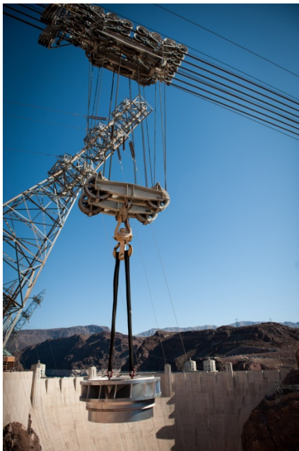
Figure 5: Installation of retrofitted turbine at Hoover Dam to provide more efficient power at a wider range of reservoir elevations.
